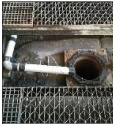
installing new service pipe
