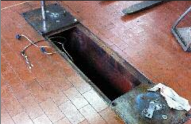
partly removed old Slift Lift
