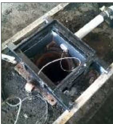
alignment and casing of the new frame
