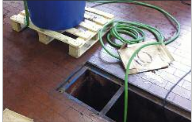
pumping-out and cleaning of the cassette interior
