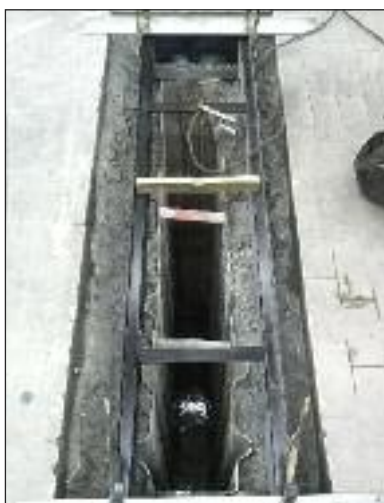
alignment before encasing new frame
