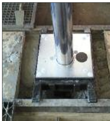
new frame encased in concrete
