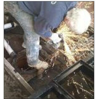
adjustment of new frame
